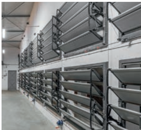
MultiVent 17 M in the gable wall for tunnel ventilation
