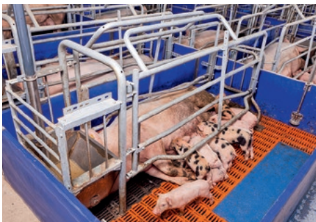
Resting area below the sow consists of cast iron slats; integrated plastic heating plate for the piglets
